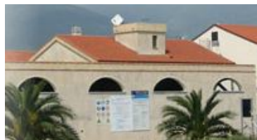
CERSAA/CCIAA headquarters (Albenga, Italy)
