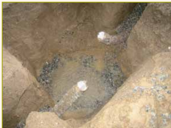
Photos 24-25. Draining tubes and prefabricated wells.
