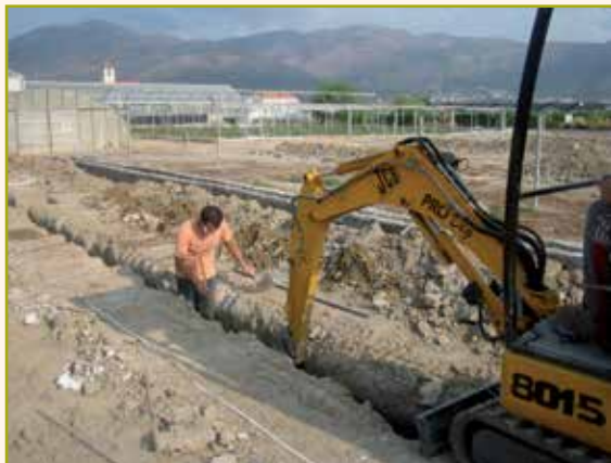
Photos 22-23. Digging of the draining system
