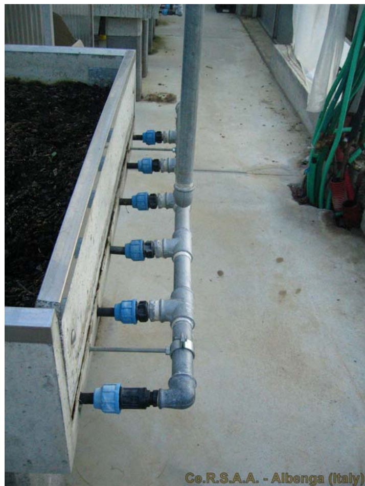
Figure 25: Pipe-heating on benches in a greenhouse in Celle Ligure (Savona, Liguria, Italy). (Source: Ce.R.S.A.A., 2010)
