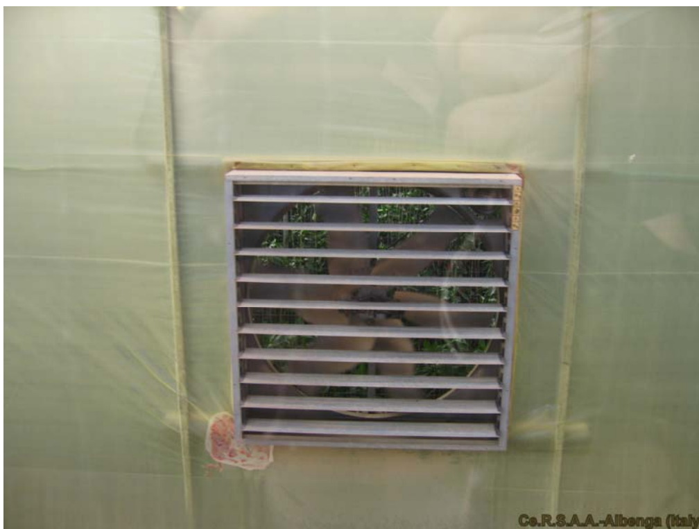
Figure 22: Air extractor for forced ventilation in a greenhouse in Murcia (Spain). (Source: Ce.R.S.A.A., 2010)
