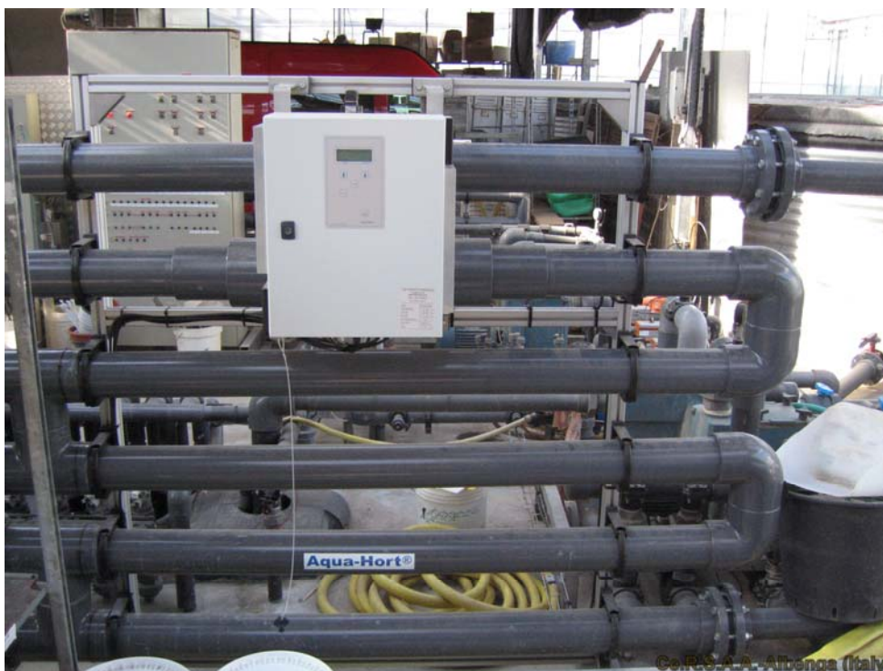
Figure 15: Disinfection system for nutrient solution recycled in a close-loop system (Frejus, Provence, France). (Ce.R.S.A.A., 2010)
