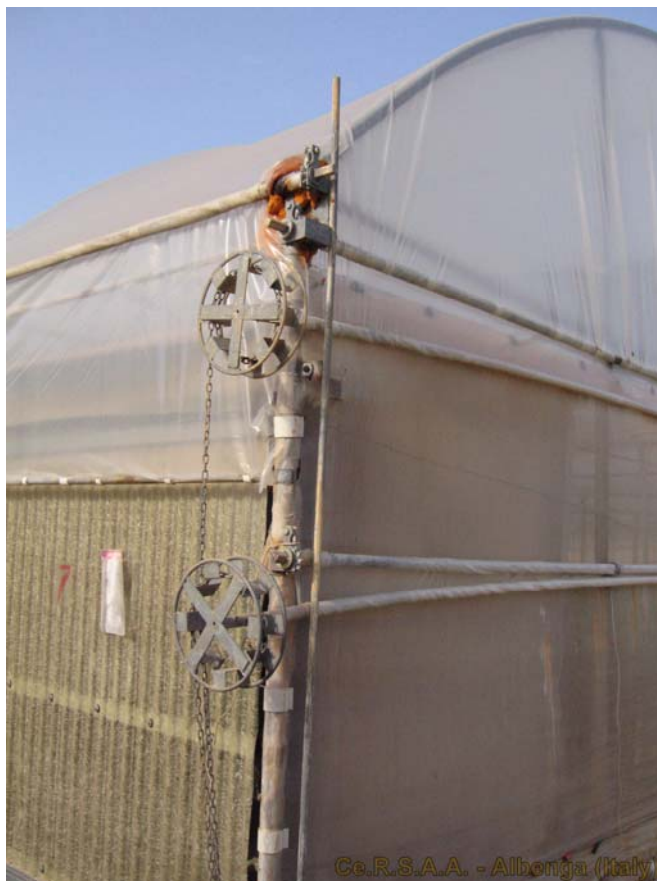
Figure 20: Device for the manual regulation of the openings (Vittoria, Sicily, Italy). (Source: Ce.R.S.A.A., 2010)
